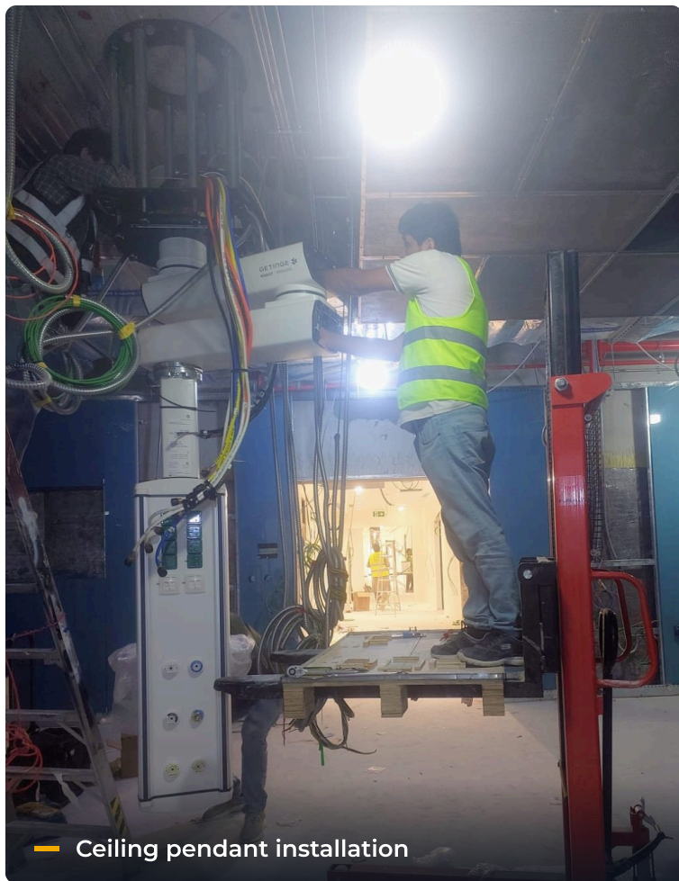
— Medical control panel installation
